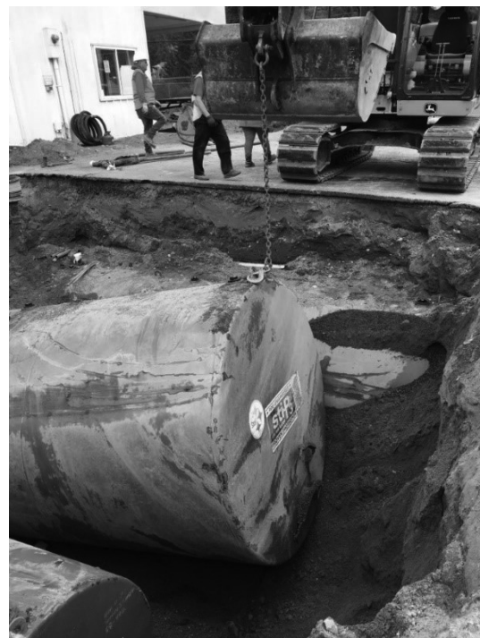
Figure 4. UST Removal
